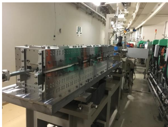
Fig. 2. Permanent dipole magnet installed in the beam transport from the booster synchrotron to the storage ring at the end of fiscal year 2017.
