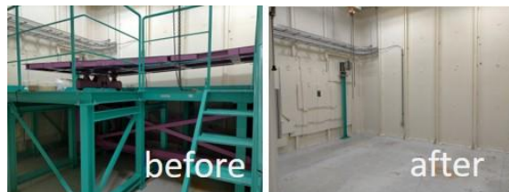
Fig. 1. Before and after the removal of the inclined stage in EH2.
