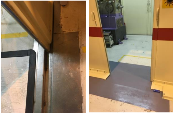
Fig. 1. Door regles of EH1 and EH3 are backfilled.
