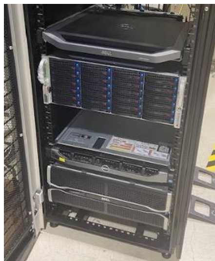
Fig. 2. New (top) and old (bottom) data storage servers in server rack.
