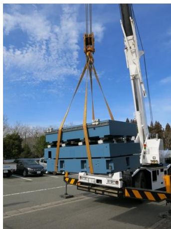
Fig. 2. Optical tables for NRS experiments were moved from BL09XU to BL35XU.
