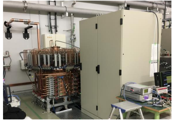
Fig. 4. New 476 MHz RF source based on solid-state amplifiers.
