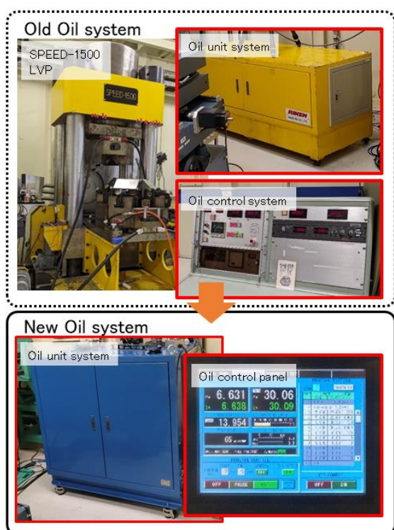
Fig. 1. Old oil system and new oil system installed at BL04B1.
