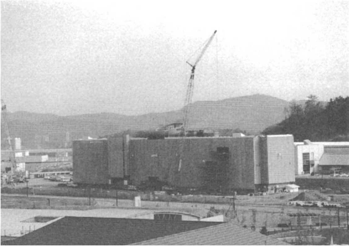
Main Building (view from the Guest House)
