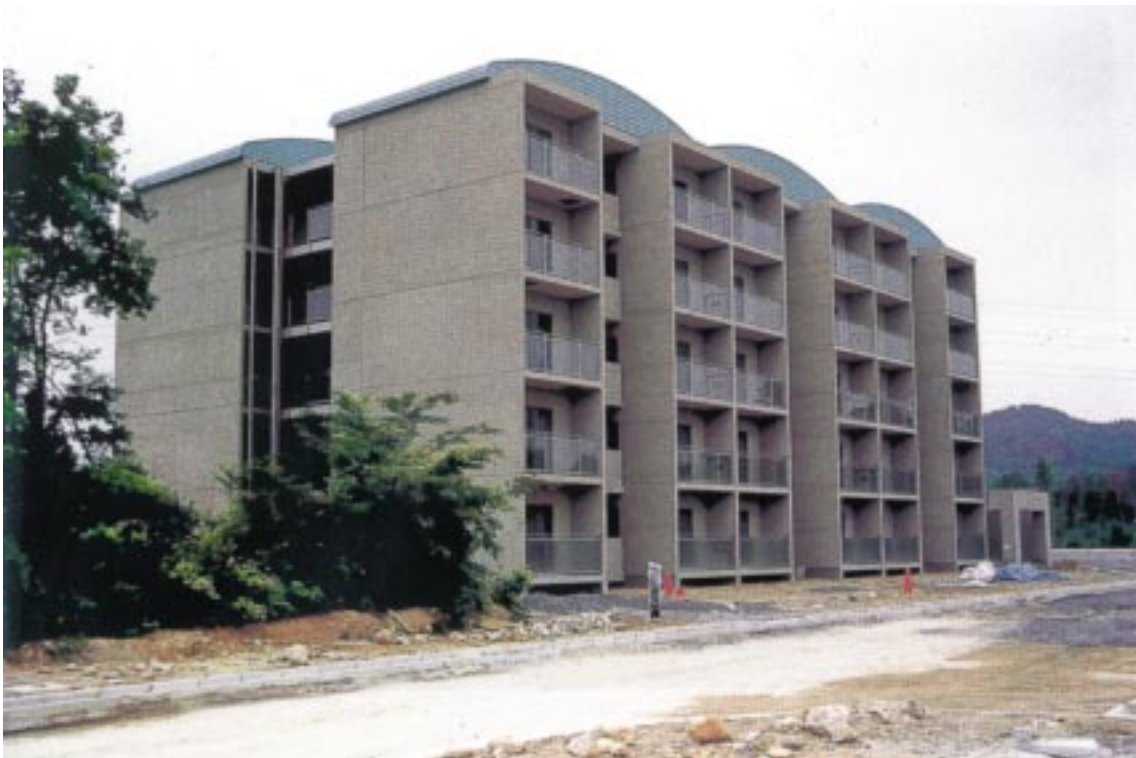
The guest house of the SPring-8 facility being made ready for welcoming guests.
