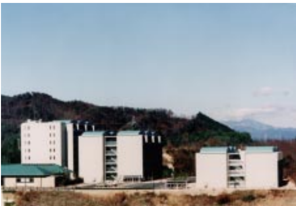
Guest House "B" "C" "D" (side view)
