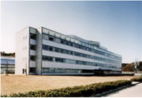
Main Building (outside view)
