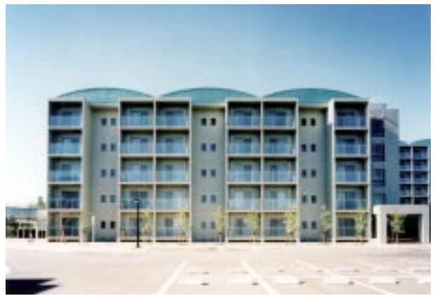
Guest House "C" (front view)
