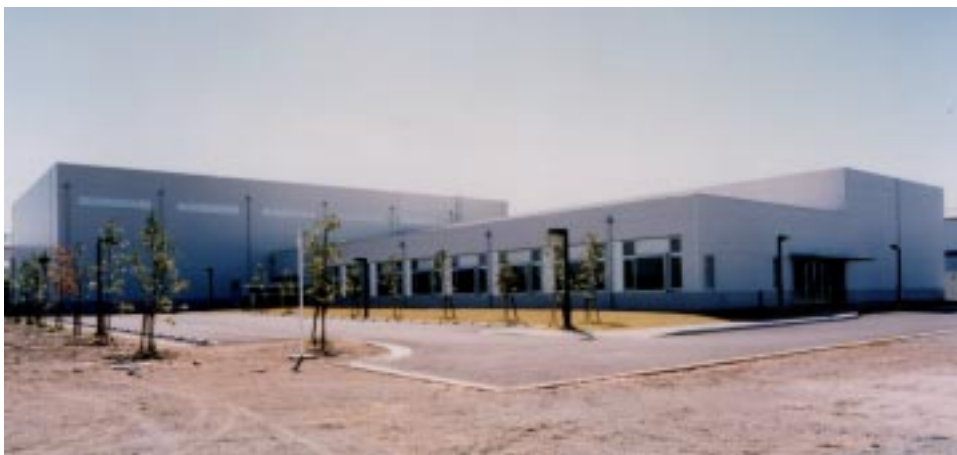
Accelerator and Beamline R&D Facility
