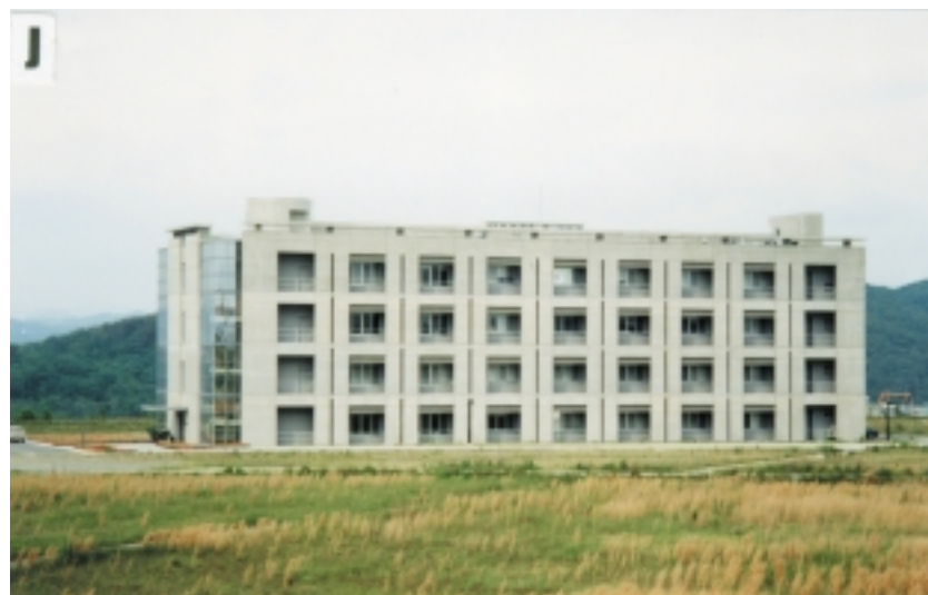
Fig. 1-3 Outward appearances of the new buildings and apparatus in 1997
