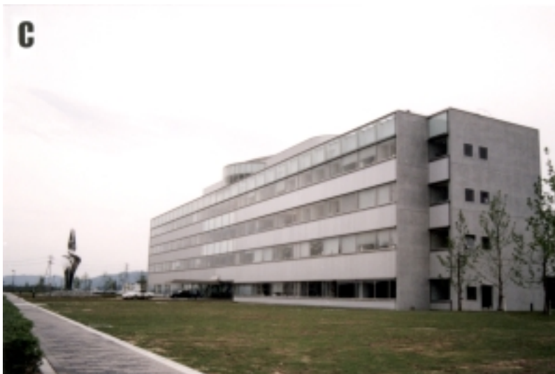
Fig. 1-1 Outward appearances of the new buildings and apparatus in 1997
