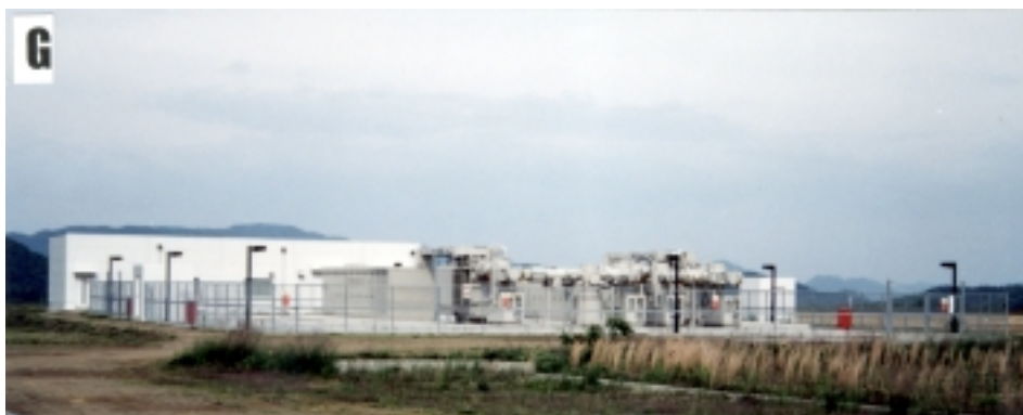
Fig. 1-2 Outward appearances of the new buildings and apparatus in 1997 D:Guest House F:Accelerator and Beamline R&D Facilities E:Machine Laboratory Extra-High Voltage Third Substation
