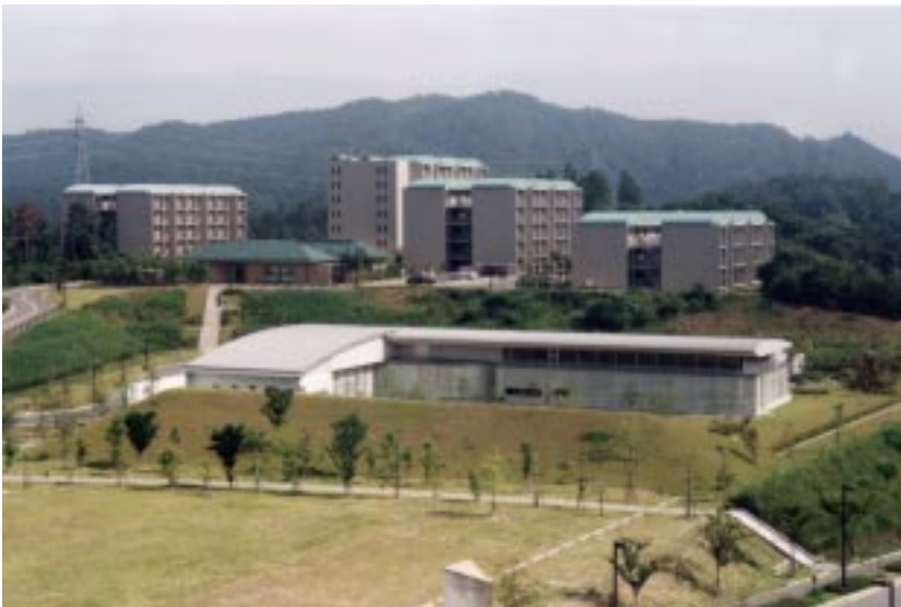
Three guest houses were constructed and opened in October. A cafeteria (in front) was opened in August.
