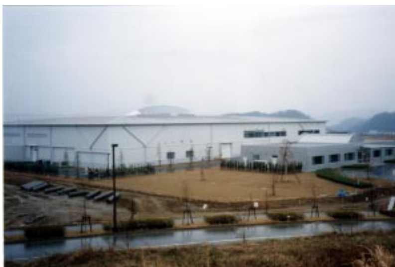
Building for New SUBARU storage ring ( E=1.5 GeV and C=118.7 m) for VUV radiation constructed by Himeji Technical Institute near the injector linac of SPring-8 facility.
