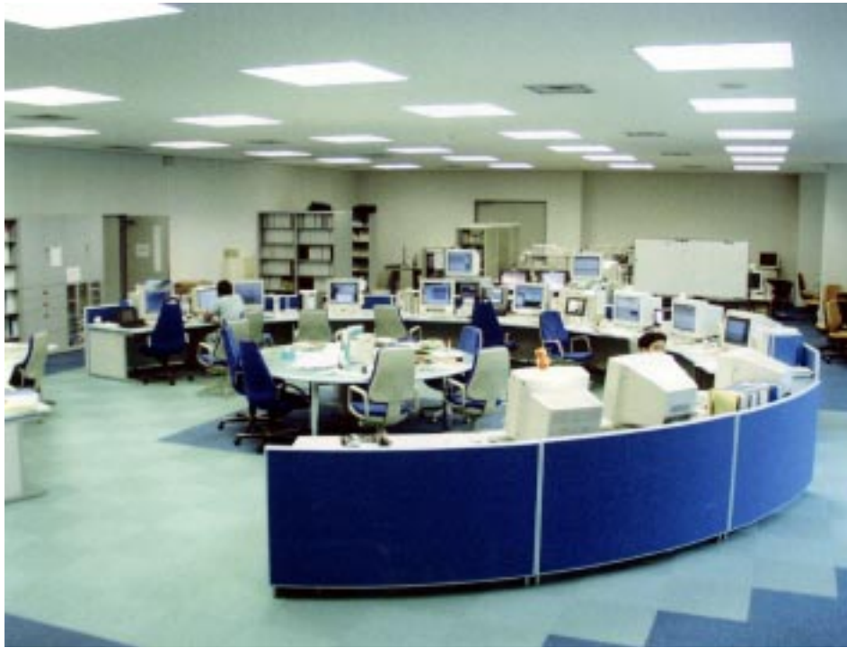
Central Control Room for machine and beamline operation, which is performed with a number of workstations on a round desk.
