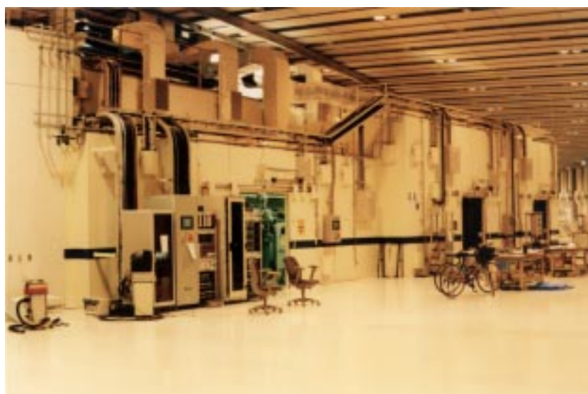
Radiation shielding hutch for high energy scattering beamline BL08W.
