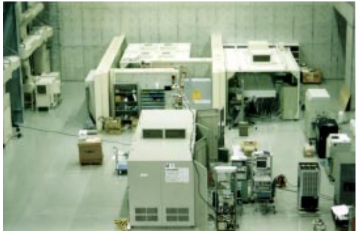
RF gun test station under construction in Machine Laboratory. A 35 MW klystron, a modulator, waveguide and laser system were installed.
