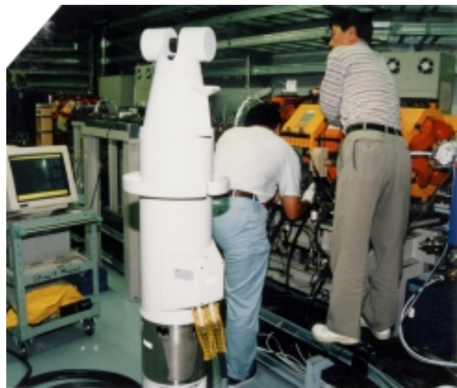
Fig. 9. Realignment of multipole magnets.
