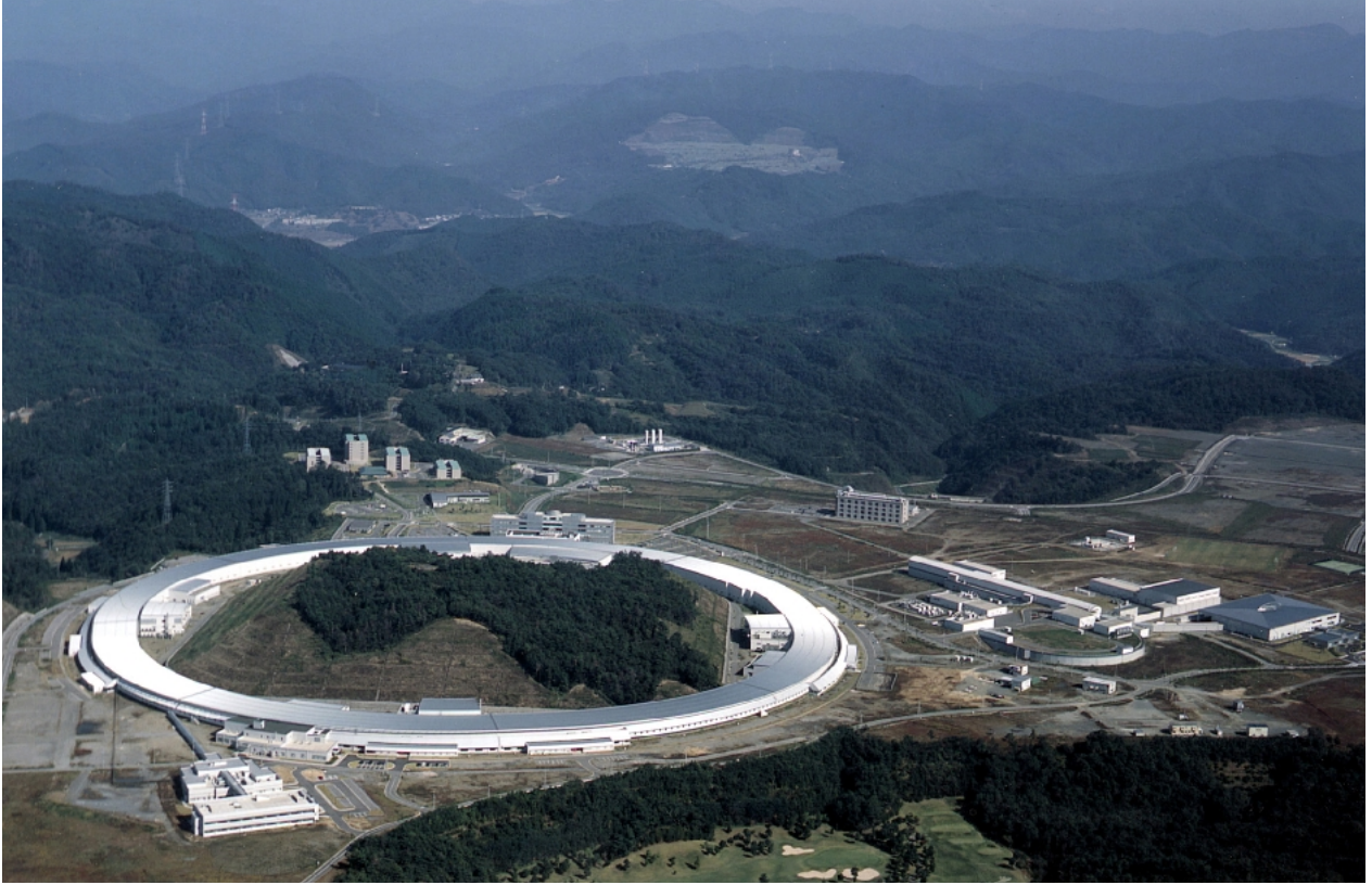
Bird's eye view of the SPring-8 facility.
