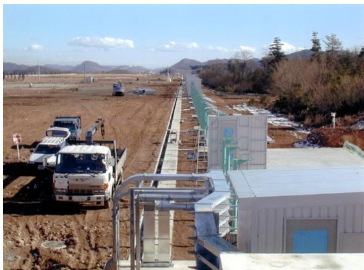
The 1-km long beamline BL29XUL under construction (as of Dec. 1999). A two-storied building for experiments is being constructed at the end of the beamline.
