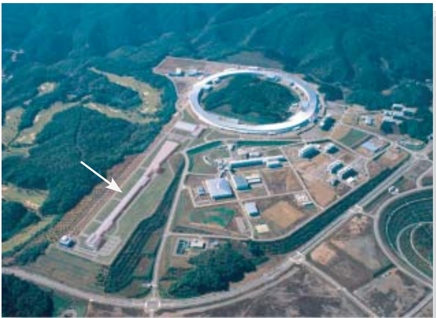
Fig. 1. Computer image of SCSS-XFEL, (left straight facility, 700 m total length), which will provide extremely intense X-ray radiation: pulsed peak power > 1 GW, pulse length < 100 fs, repetition rate 60 pps. The designated wavelength is 1 Å at 8 GeV electron beam energy. The large circular building is the existing 8 GeV synchrotron radiation facility (500 m in diameter).
