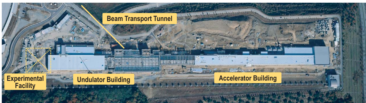
Fig. 10. Aerial photograph of XFEL construction site taken in November 2008.
