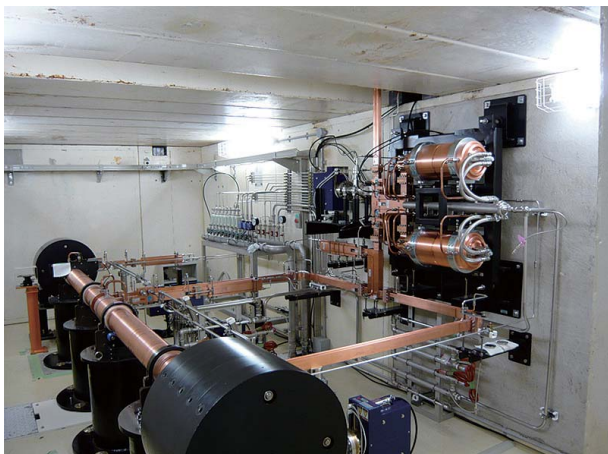
Fig. 2. Test bunker for high-power rf components.
