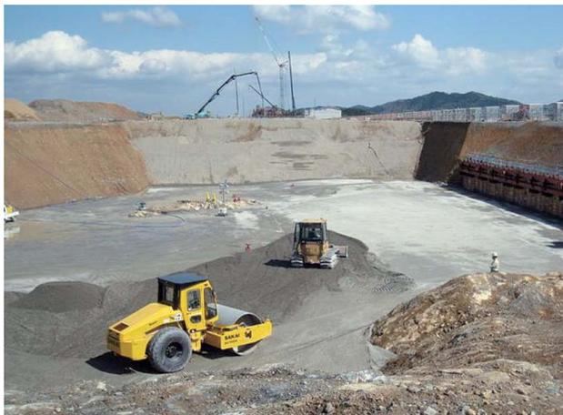
Fig. 11. Rolling procedure for forming stable and high-density artificial rock bed.
