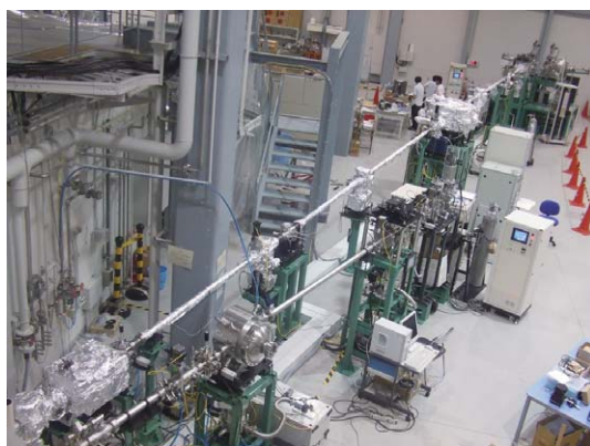
Fig. 1. Constructed high-resolution beamline BL-5 for soft X-ray spectroscopy analysis of Industrial Materials.
