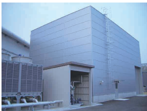
Fig. 2. Photograph of the LEPS2 experimental building. This building was constructed by the support of the RIKEN Nishina Center. A cooling system for the magnet coil is also seen in front of the LEPS2 building.
