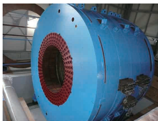
Fig. 4. Photograph of the E949 solenoid magnet installed in the LEPS2 experimental building. The diameter of the magnet yoke is 5 m and the length is 3.5 m. It is placed in the pit with the depth of 1.5 m.
