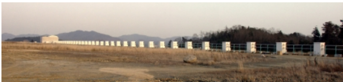
Fig. 4. A section of transport channel of the 1 km beamline (BL29XU) in open air.
