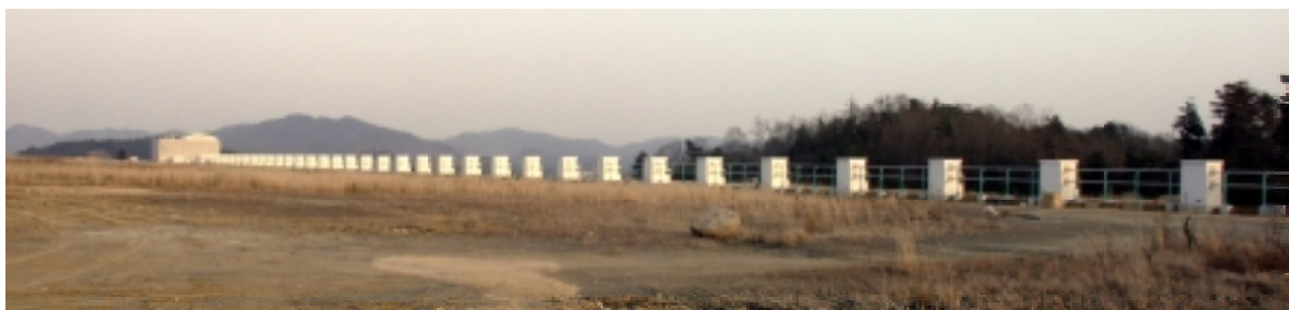
Fig. 4. A section of transport channel of the 1 km beamline (BL29XU) in open air.
