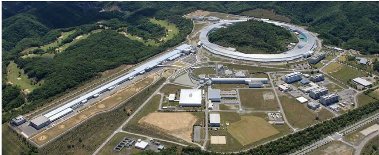
Figure 5.1: SPring-8 Accelerator Complex; SPring-8 (right top) and SACLA (left).
